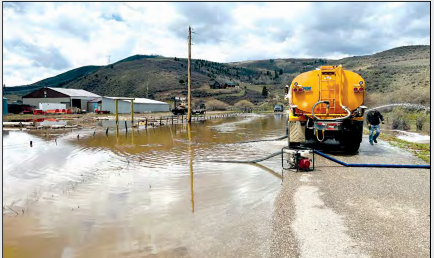
County employees pump water across Fairview South on Monday, following flooding on the south side of the road. As the record snowpack melts, flooding concerns remain high. Visit SVInews.com and listen to SVI Radio for the latest flood forecast. SVI PHOTO/DUKE DANCE
