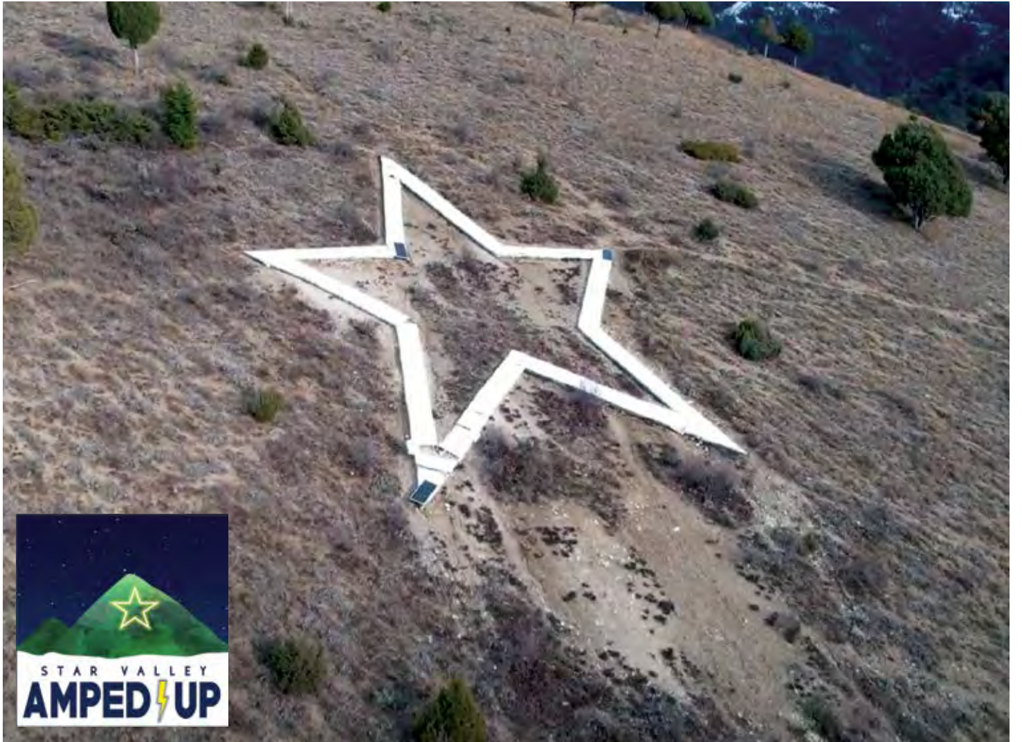
The current structure of the Star includes aluminum with solar panels. The panels have not been reliable and the aluminum has not held up well over the past few years. COURTESY PHOTO/TOWN OF AFTON
